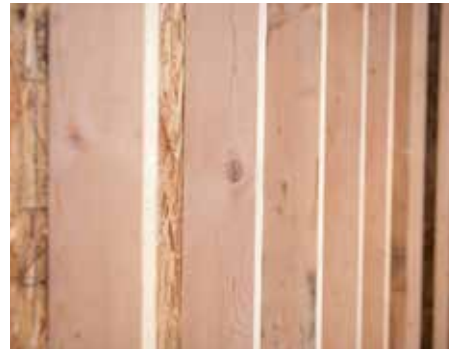
2" x 6" exterior studs on 16" center
