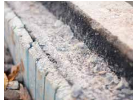
Foundation walls 10" poured 4,000 pound concrete with 1/2" rebar
