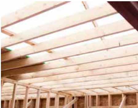
2" x 6" rafters on 16" center or trusses
