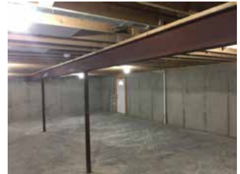
2" x 10" floor joists on 16" center and Steel I-beams
