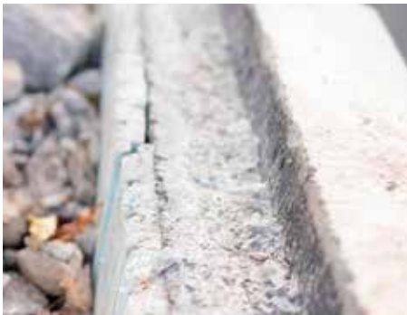
Foundation walls back filled with crushed stone
