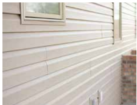
Vinyl siding on non-brick areas
