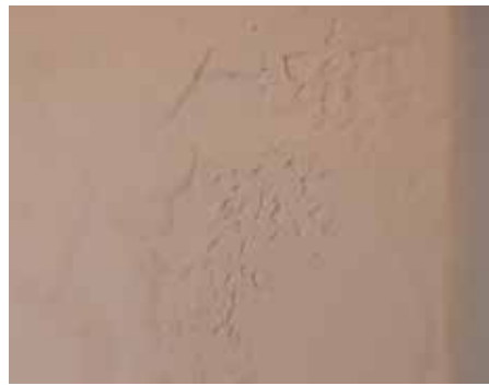
Hard-coat plaster with textured finish
