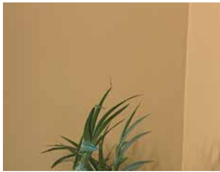
Smooth plastered walls in kitchen and bathrooms
