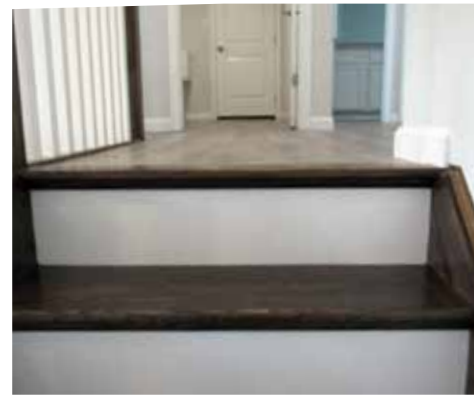
Stairs Painted Riser
