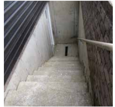
Exterior Basement Steps
