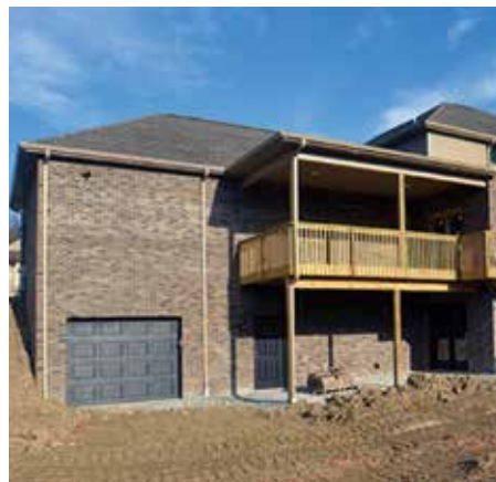
Excavate Under Garage
