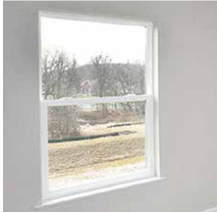
Casement Single Hung Window with Plaster Return
