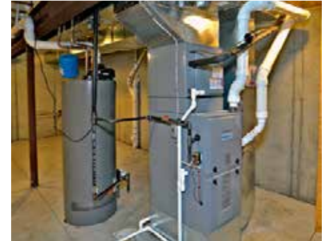
95% High efficiency gas furnace with add on humidifier (10yr warranty - parts & labor)
