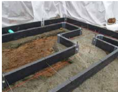
Form-a-drain with stone back fill
