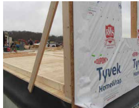
7/16" OSB board exterior walls
