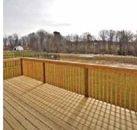
Uncovered Wood Deck
