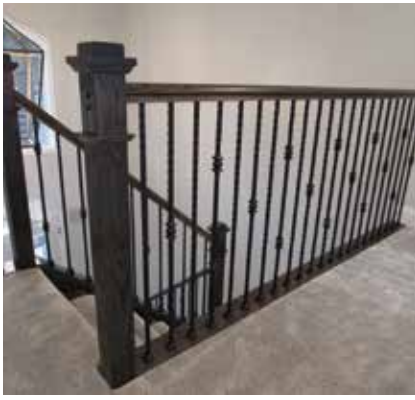
Wrought Iron Railing
