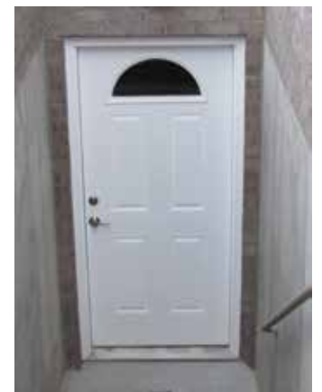
Single Basement Exit Door
