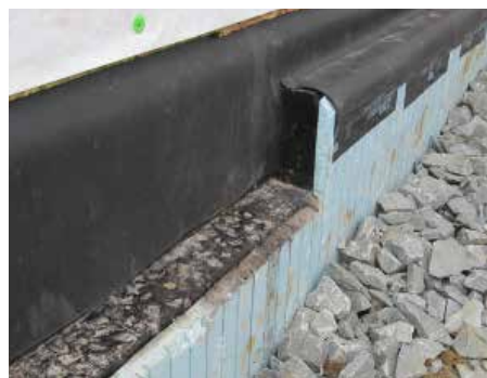
16" rubber water flashing behind brick
