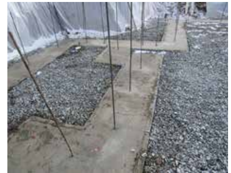
20" poured 4,000 concrete footer with rebar (RWS does not use gravel footers)
